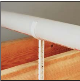
Support horizontal runs of vent pipe in the attic.
