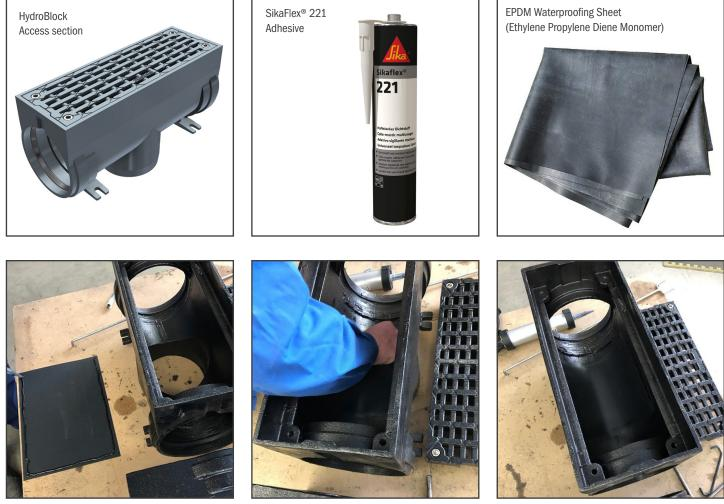
Prepare surfaces, making sure the channel is free of dust/dirt/grease/oil/etc. Cut waterproofing sheet to cover at least 2" beyond the outlet on all sides. Apply a 1/4" bead of *SikaFlex 221 Multi-Purpose Adhesive* 1" inside the edge of the waterproofing sheet.
