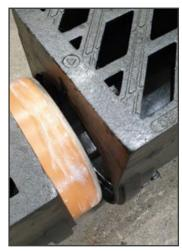
Align the socket of the second section and push the two sections together as far as possible.
