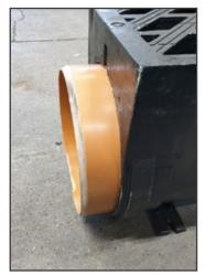
Insert the pipe connector\* into the socket end of the HydroBlock section.
