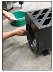
To facilitate installation, apply pipe joint lubricant to the pipe connector (OD) and the rubber seal inside the HydroBlock section.
