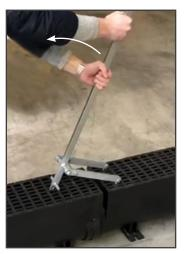
Using the HydroBlock installation tool\*, pull the two sections together firmly
