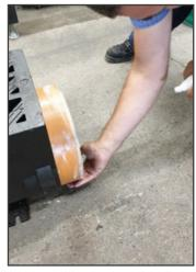
Lay the section horizontally on the feet and lubricate the exposed OD of the pipe connector, and rubber seal inside the second HydroBlock section
