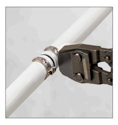
2. Close clamp ear with ratchet pincer tool. Tool will not release until clamp is fully closed. Remove any defective connections. Test all completed joints.
