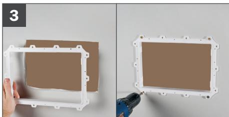
Insert frame, with elongated lip facing inward, into hole and screw the frame to the wallboard through provided holes. Insert as shown.
