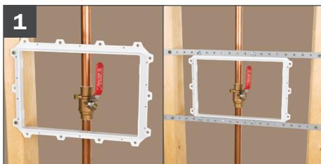
Hang the frame, with elongated lip facing outward, on support bars or directly to studs. Level and secure around device/application needing future access and service.
