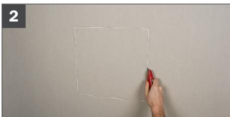
Level frame, trace, remove frame and cut hole.
