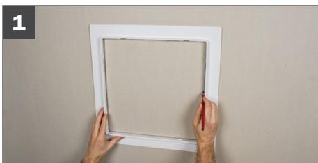
Use frame as a template to cut the access hole.
