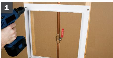
Hang the frame on support bars or directly to studs. Level and secure around device/application needing future access and service.
