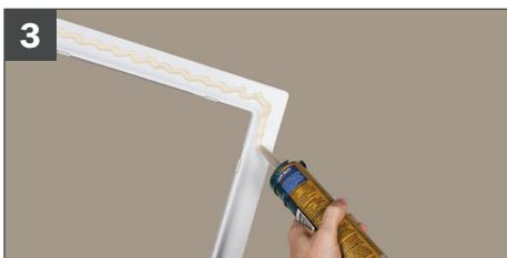
Apply a bead of adhesive around perimeter of frame and insert as shown. Remove excess adhesive.
