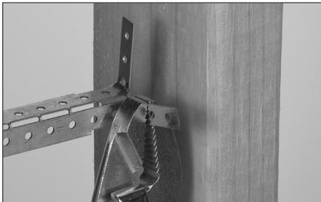
Bend in both tabs to fit the bracket inside the stud bay.
