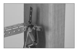
Bend in both tabs to fit the bracket inside the stud bay.
