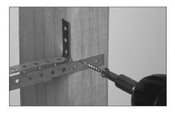
Use screws or nails to secure bracket to either the front or inside of stud.
