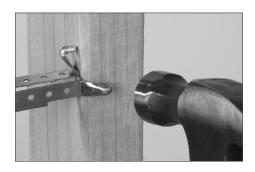
Edge brackets are also offered with self-nailing barbs that can be driven directly into wood studs.
