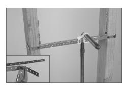
If stud bay is not wide enough, tear perforation on the vortex of the bracket to best fit the opening.
